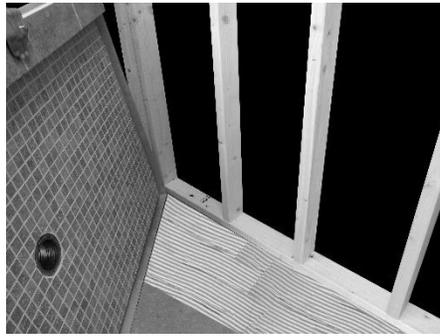
2. Maneuver a back corner of the tray into the back left (or right) corner of the rough opening.
