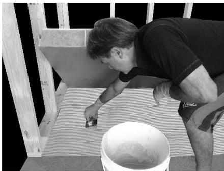
5. Apply thin-set mortar cement to the front half of the sub-floor area while ensuring the tray remains securely supported (by a second person, your shoulder, etc.).
