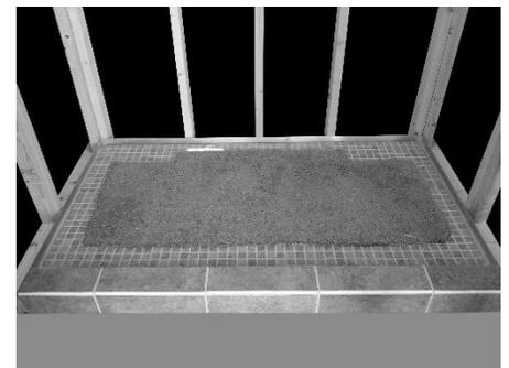
9. Clean any excess cement protruding from the front edge of the tray. Cover tray with protective material before proceeding with further construction or installation activities.
