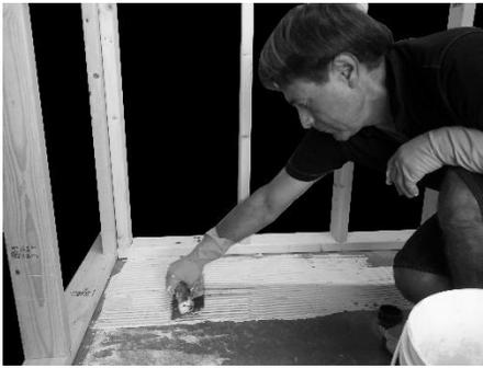
1. Evenly apply thin-set mortar cement to sub-floor area across the back of the rough opening.
