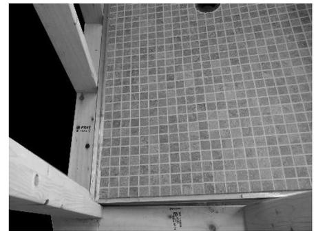
6. Ensure drain pipe slots into, and is centered within, the drain body and lower tray into final position (see note below).
