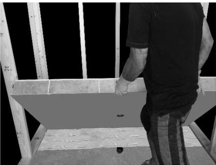
4. Begin to lower tray, adjusting as required to maintain a tight fit with the back of the rough opening.
