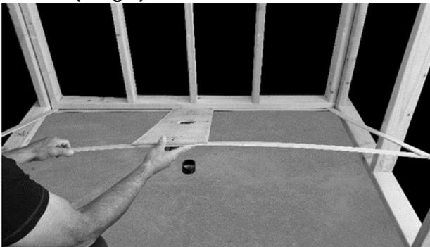
3. Lower tray template slowly. Do not bend or force template into position. Check that studs do not protrude into space and obstruct the template as it is being lowered
